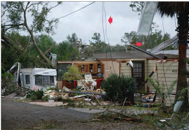
FIGURE 23-2 Check the scene for dangers that could threaten your safety or the safety of others, such as downed wires and unstable structures.
